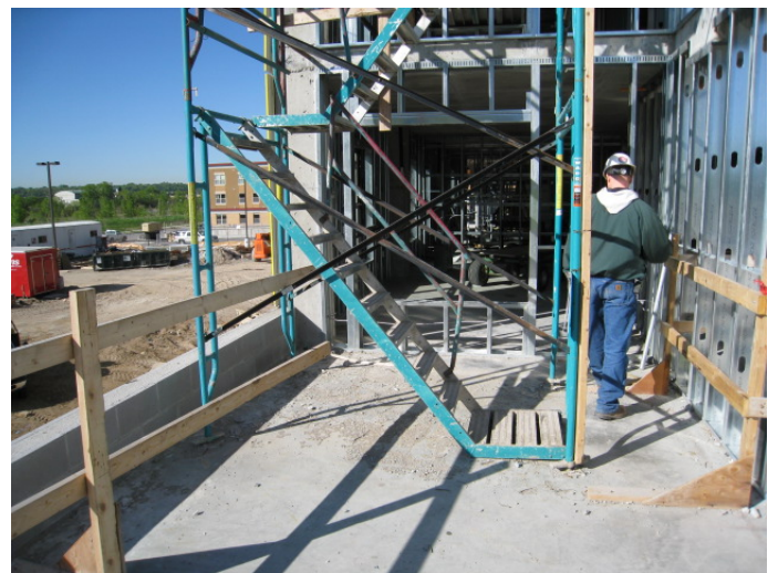
Stairway access on a scaffold
